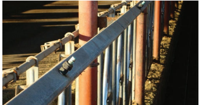
Square tubing can be used for soaker line
