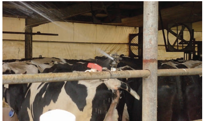
High capacity soaker nozzle on side of holding pen
