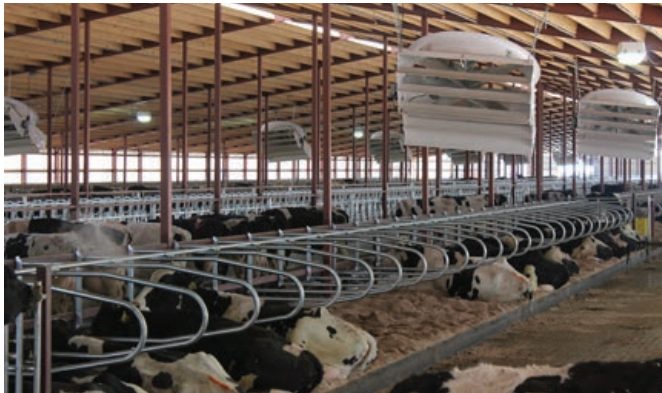
Fans properly spaced to provide effective cow velocity to prevent heat stress
