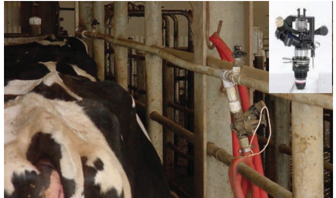
High capacity soaker nozzle mounted on the side of holding pen and RainBird low angle nozzle.
