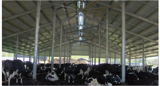
Overhead high volume/low speed and low volume/low speed fans may fail to provide adequate ECV. Photo compliments of Dr. Jeffery Bewley, University of Kentucky.
