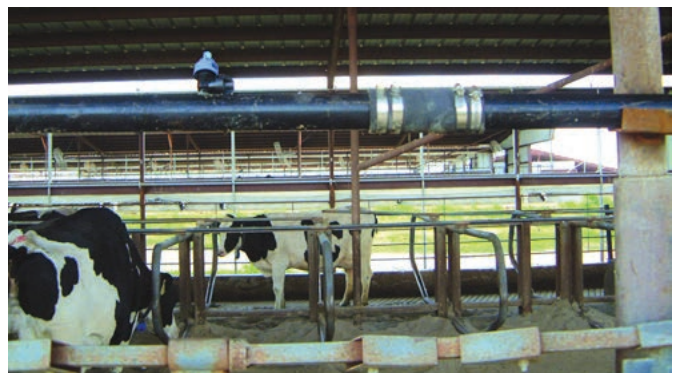
Steel pipe coupled with radiator hose
