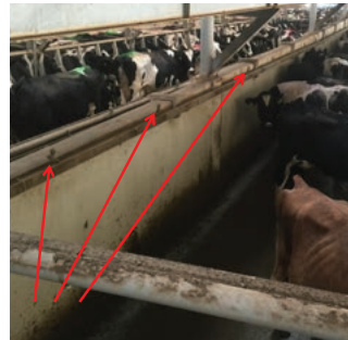
(Left) Tee-jet nozzles along cow platform in the parlor for soaking after milking. Rapid exit goes up, there is a 10 second delay to allow time for cows to step out, and the soaker line is activated for 1.5 to 2 minutes. Soakers are set on 6 foot centers on the cow platform.
