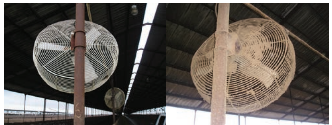
Maintaining clean fans is critical for both air velocity (ECV) and efficiency
