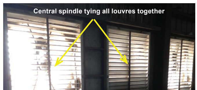
Check louvres, especially in cold weather. Decouple bottom louvre during winter because of freezing shut. If freezing occurs, all louvres will be in closed position when fans are turned on.
