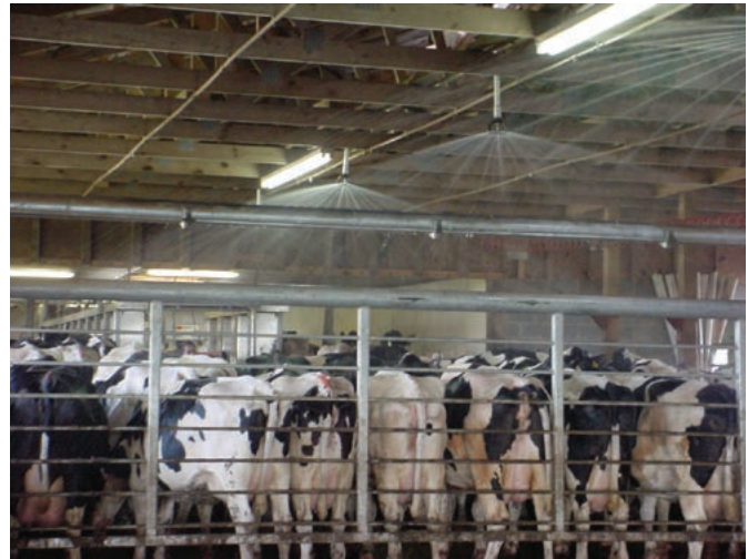
Senninger Super Spray nozzle in the grid soaker system in holding pens
