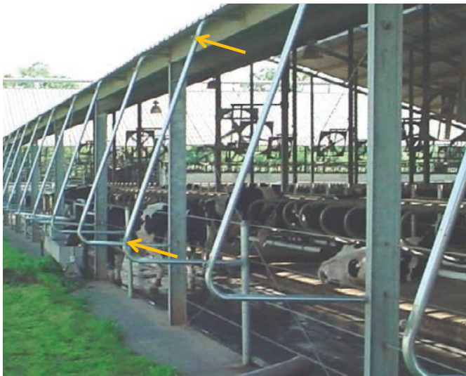
Perlins for attaching shade cloth to north to south oriented barns. Arrows indicate eye bolts for running cables to attach shade cloth.
