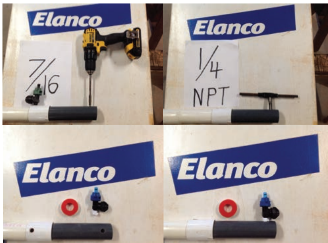
Installation of nozzle body into PVC pipe
