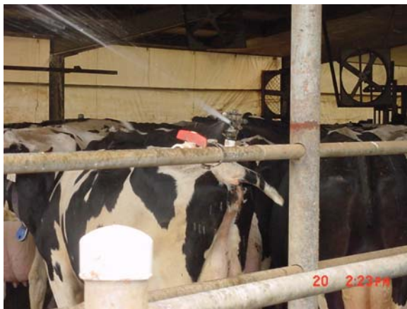
Rain Bird 2045-PJ low angle nozzle
