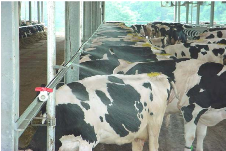
1 ½ " PVC with threaded TeeJet Nozzle body mounted to angle iron bracket
