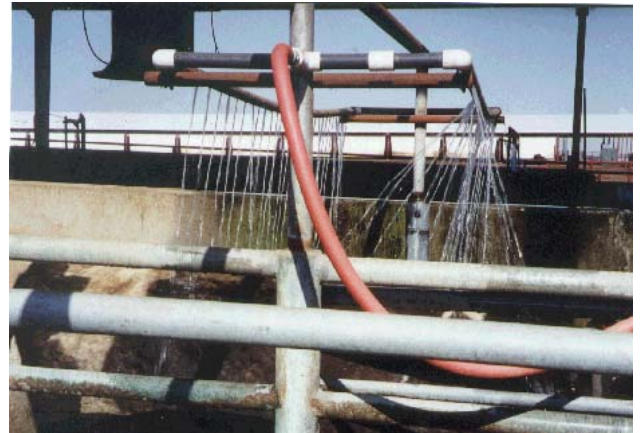
PVC Pipe with holes drilled for shower
